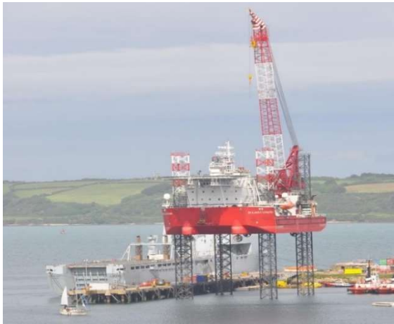
G: Seajacks Leviathan jacked up on Queens Wharf
