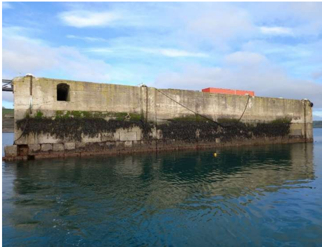
A: Northern Arm Concrete structure, looking north
