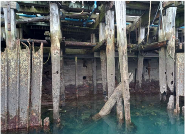
D: Western Wharf Condition of Timber Piles, looking west
