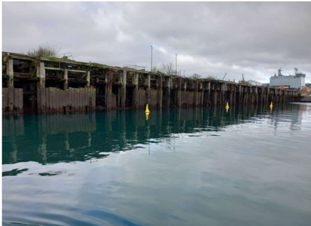
C: Western Wharf, looking northwest
